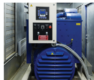
Automatic standby generator
